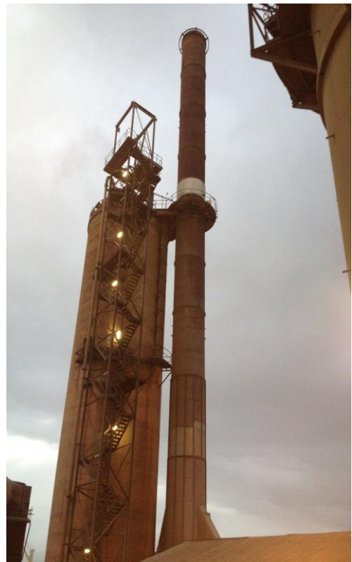
Figure 1: Kiln 4 Main Stack (RP 4A)
