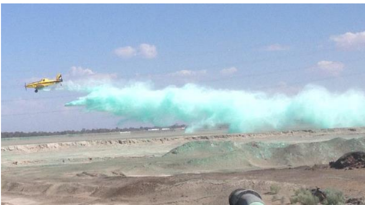
Aerial application of dust suppressant
