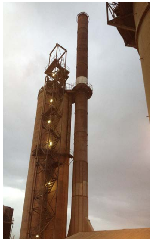
Figure 1: Kiln 4 Main Stack (RP 4A)
