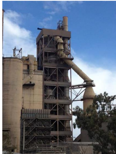
Pre-Calcliner Plant Stack (Stack 4B)
