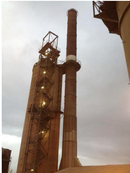
Dry Process Kiln Stack (Stack 4A)
