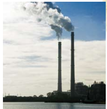
Torrens Island Power Station. Photo: Tim Lubcke
