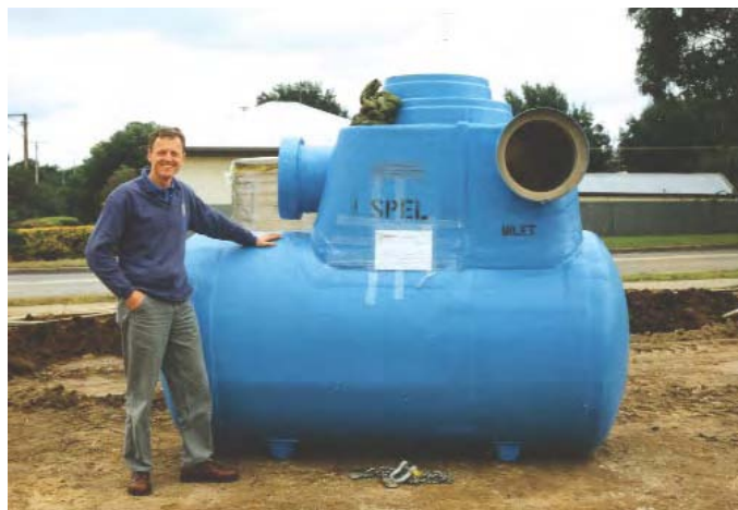
Figure 31 Manufactured unit ready for in-ground installation
