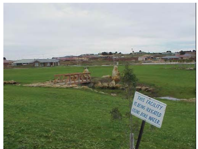
Figure 26 Large shallow basin incorporating swales
