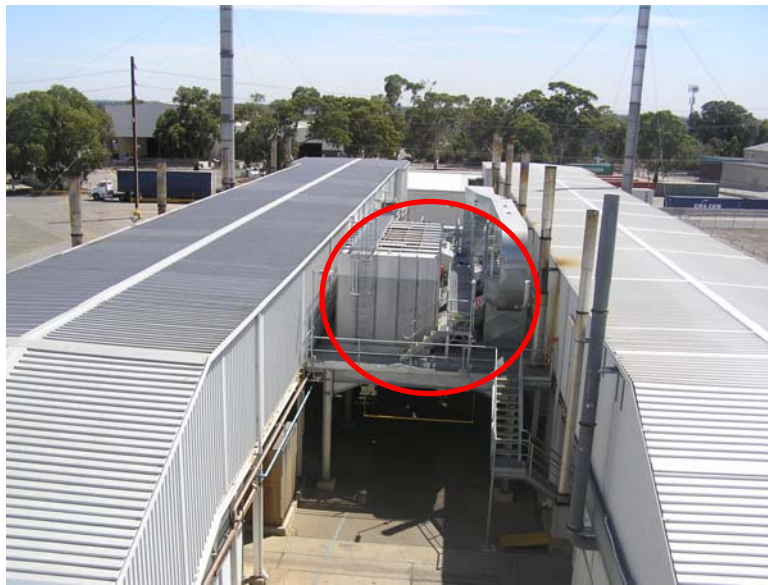
Figure 5 The thermal oxidizer with regenerative heat exchanger at Mitsubishi
