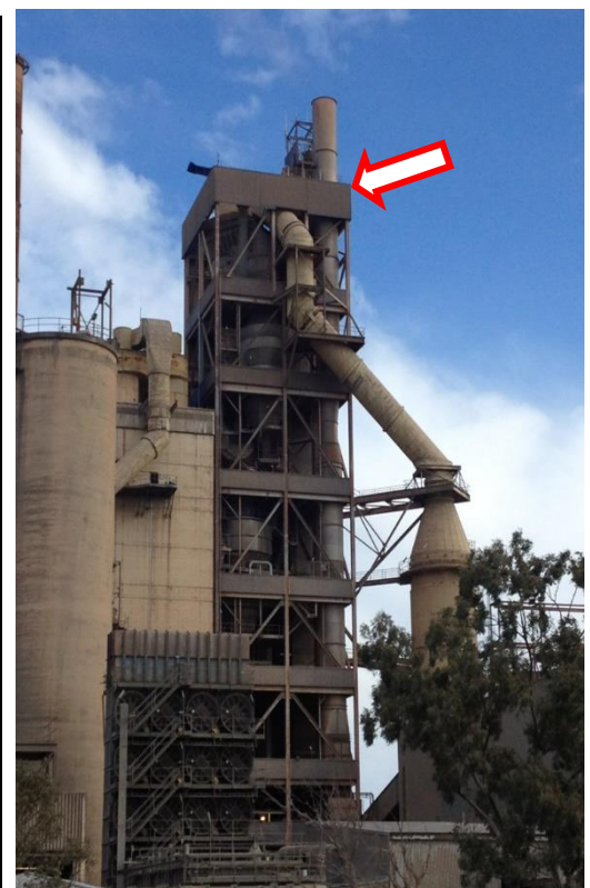
Figure 2: Precaliner Plant Stack (RP 4B)
