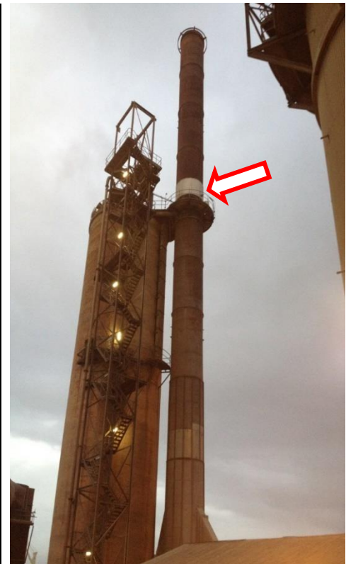
Figure 1: Kiln 4 Main Stack (RP 4A)
