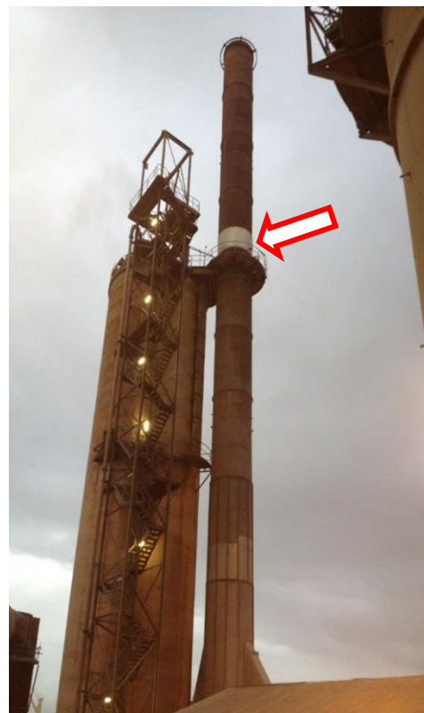
Figure 1: Kiln 4 Main Stack (RP 4A)
