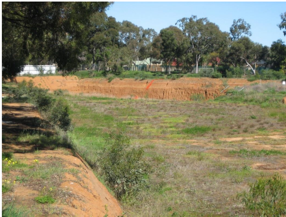
Plate 4 Remediated soils at MTS, August 2011
