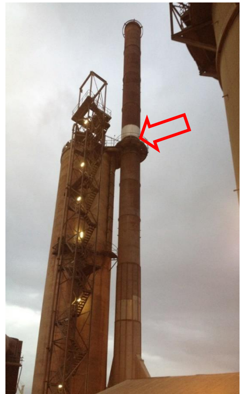
Figure 1: Kiln 4 Main Stack (RP 4A)
