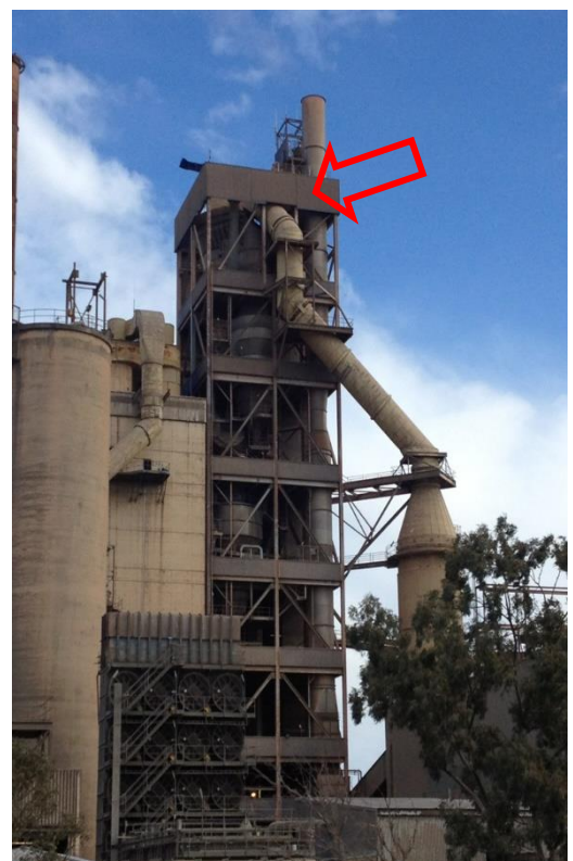
Figure 2: Precalciner Plant Stack (RP 4B)
