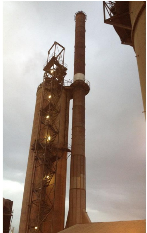
Figure 1: Kiln 4 Main Stack (RP 4A)
