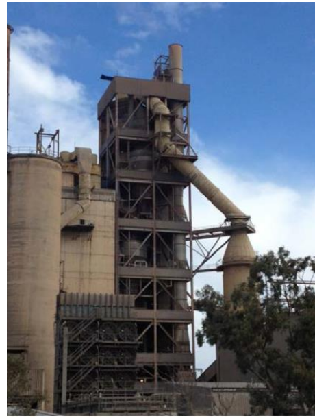
Pre-Claciner Plant Stack (Stack 4B)
