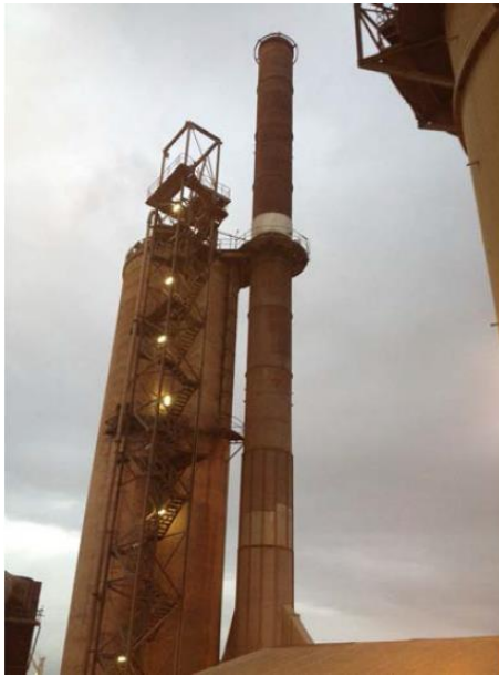
Dry Process Kiln Stack (Stack 4A)
