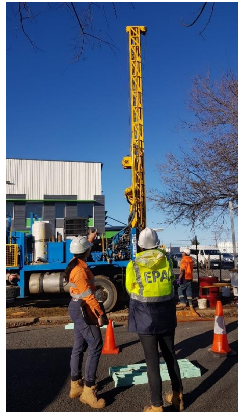
Drilling a groundwater monitoring well
