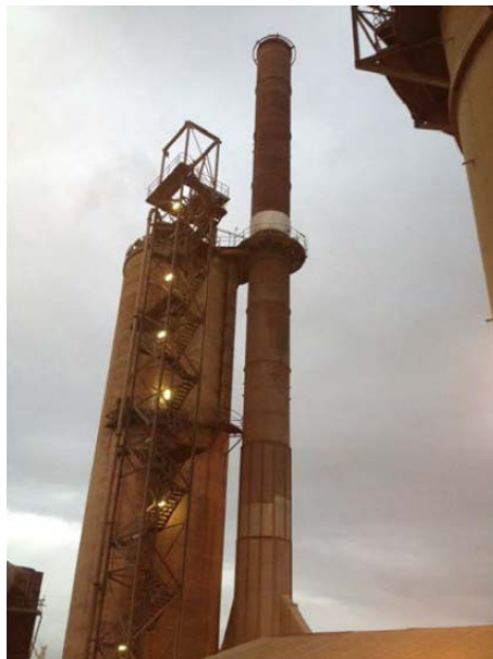
Dry Process Kiln Stack (Stack 4A)
