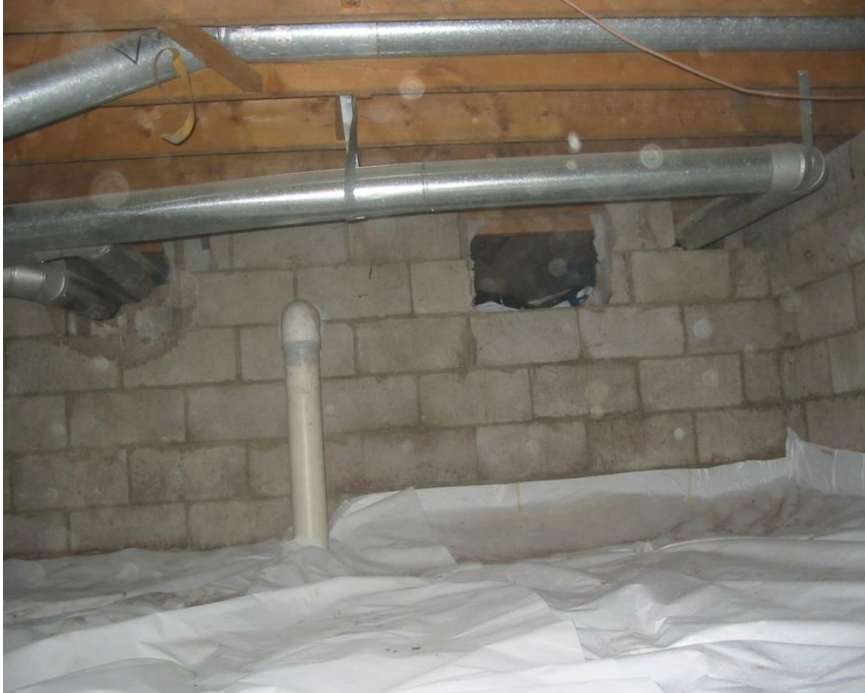
Submembrane Depressurization Layfield EL-20 (20 mil)
