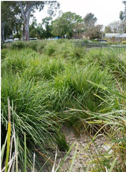
Established bio-filtration rain garden beds at Linde Reserve, Stepney
