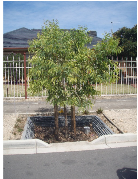
Tree pit bio-filtration system, Beechway Ave, Brooklyn Park
